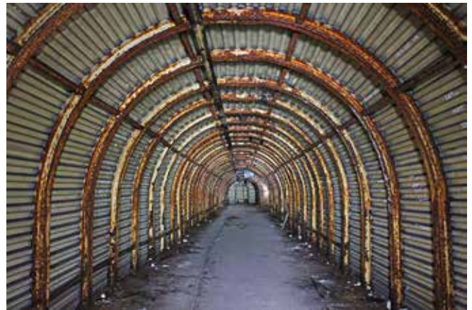
Tunnel after clearance of rubble and rubbish.
